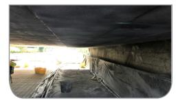
A sprayed concrete overlay was required to the deck soffit of Fulney Bridge, Spalding to contain two newly installed Impressed Current Cathodic Protection (ICCP) systems adjacent to the two half joints to a depth of 30mm, and also to distribute the ICCP current.
